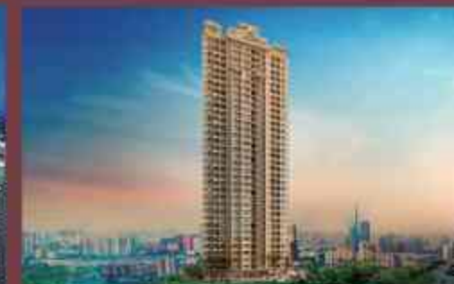
SAI PLATINUM KHARGHAR
