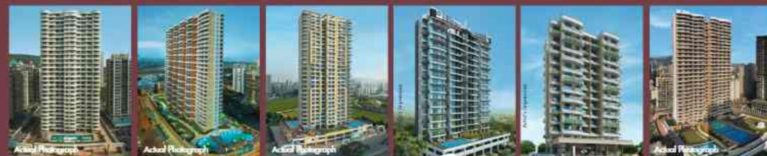
SAI SPRING KHARGHAR G+29 Storeyed Tower
