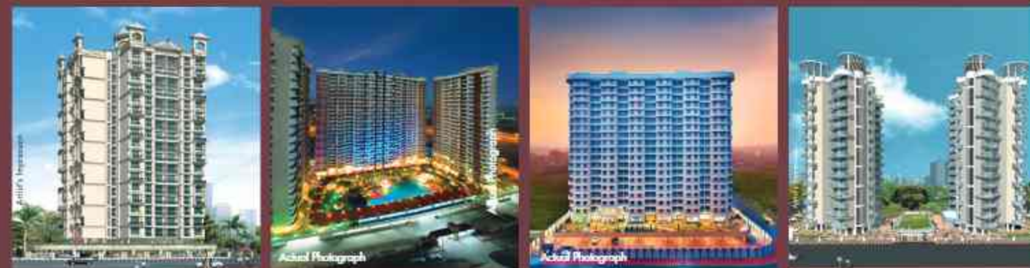
SAI JEWEL KHARGHAR G+18 Storeyed Tower
